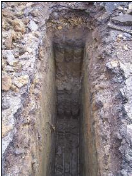
Figure 10: Deep test pit
