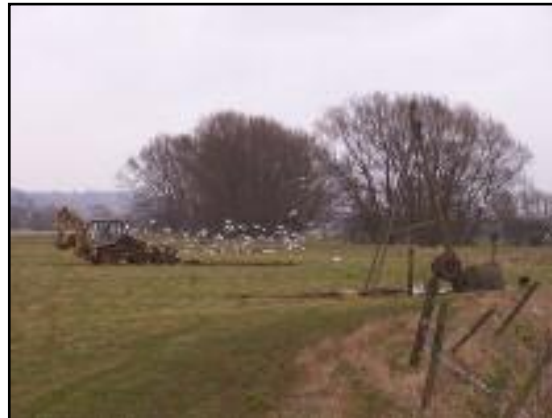
Figure 1: JCB excavating test pit and cable percussion rig in foreground.
