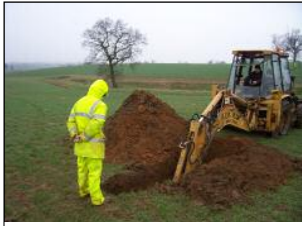
Figure 8: Engineer supervising test pit excavation.
