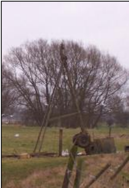
Figure 4: Cable Percussive Boring Rig
