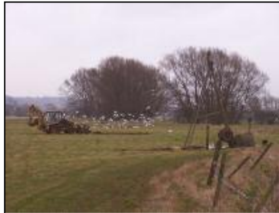
Figure 1: JCB excavating test pit and cable percussion rig in foreground.
