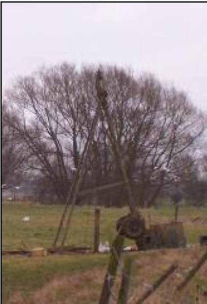
Figure 4: Cable Percussive Boring Rig
